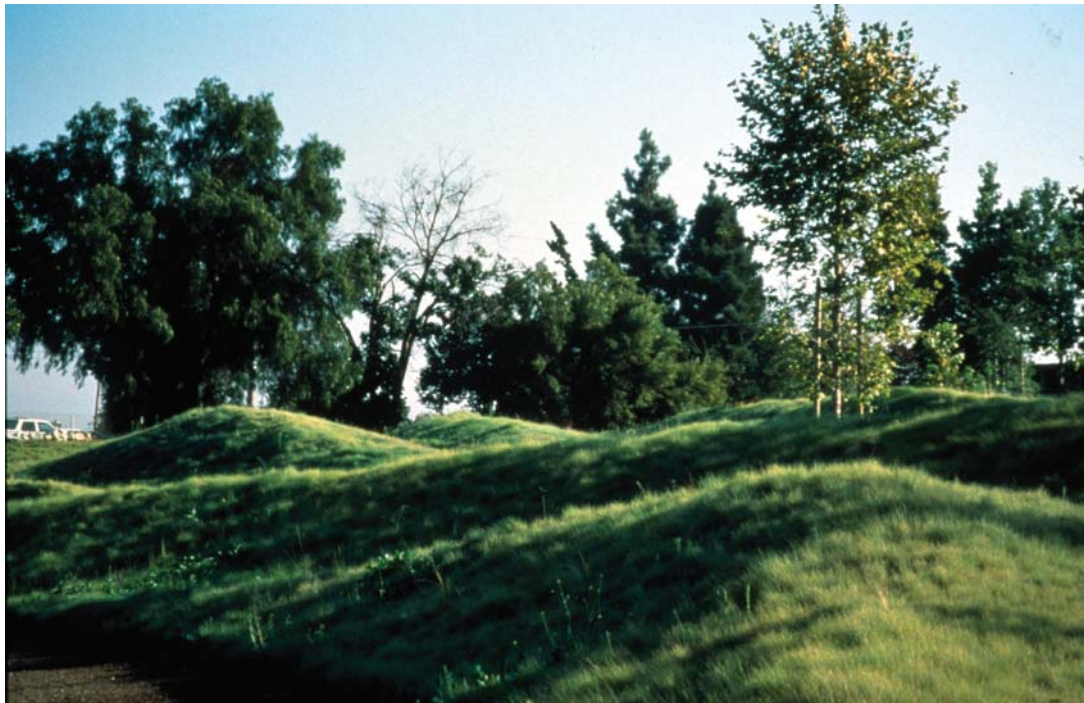
BERMING FOR NOISE MITIGATION
